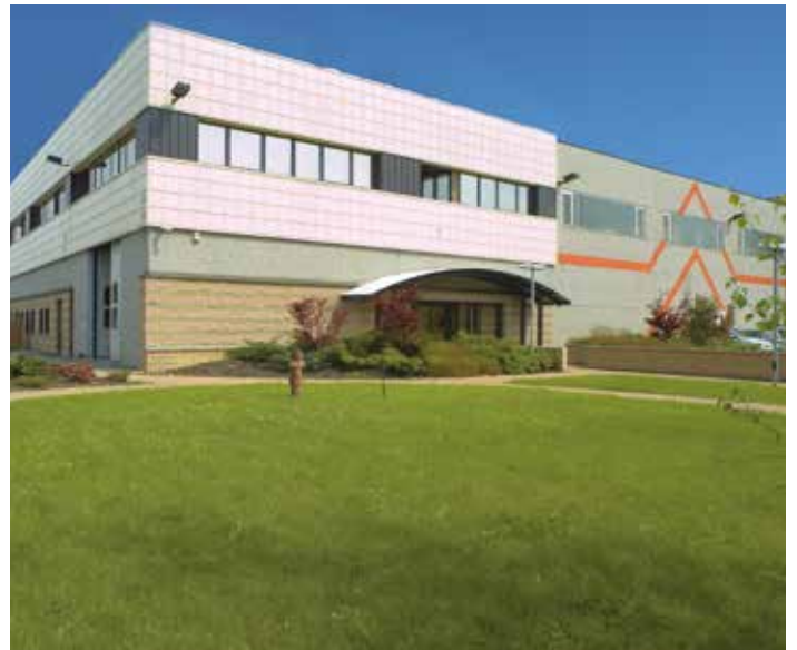
Production site, Sizzano (PV)
